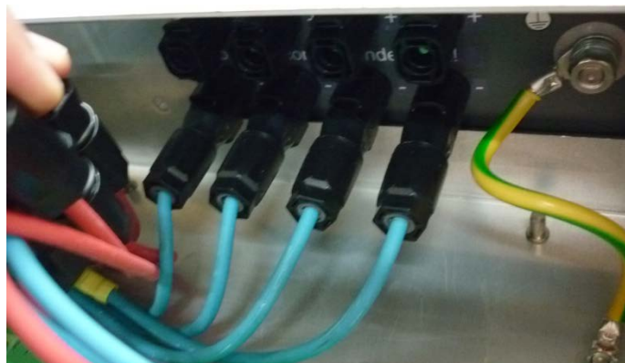
Fig. 31: Create Sunclix connectors
